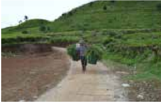
Repairs to Cibadak and Baru Mekar roads in Margaluyu village. 400m x 2m.
